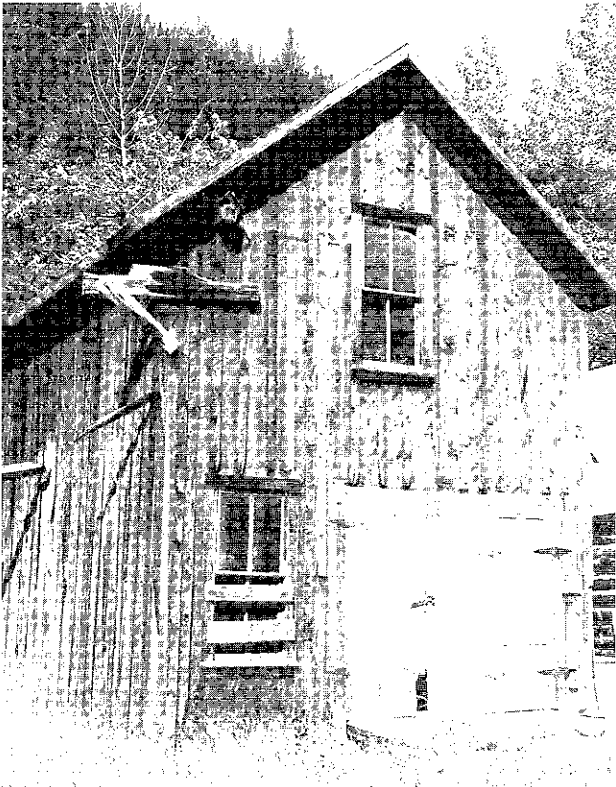
A typical structure at Rimini.
